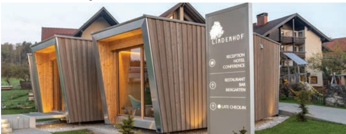
The reception in front of the Lindenhof - in modern Mohab mini-houses
